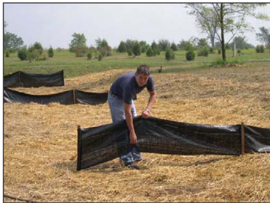
Improperly installed siltation fence in the tri-county area
