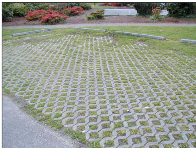
Pervious pavement for stormwater infiltration
