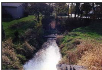
Exposed sewer pipe from stream downcutting
