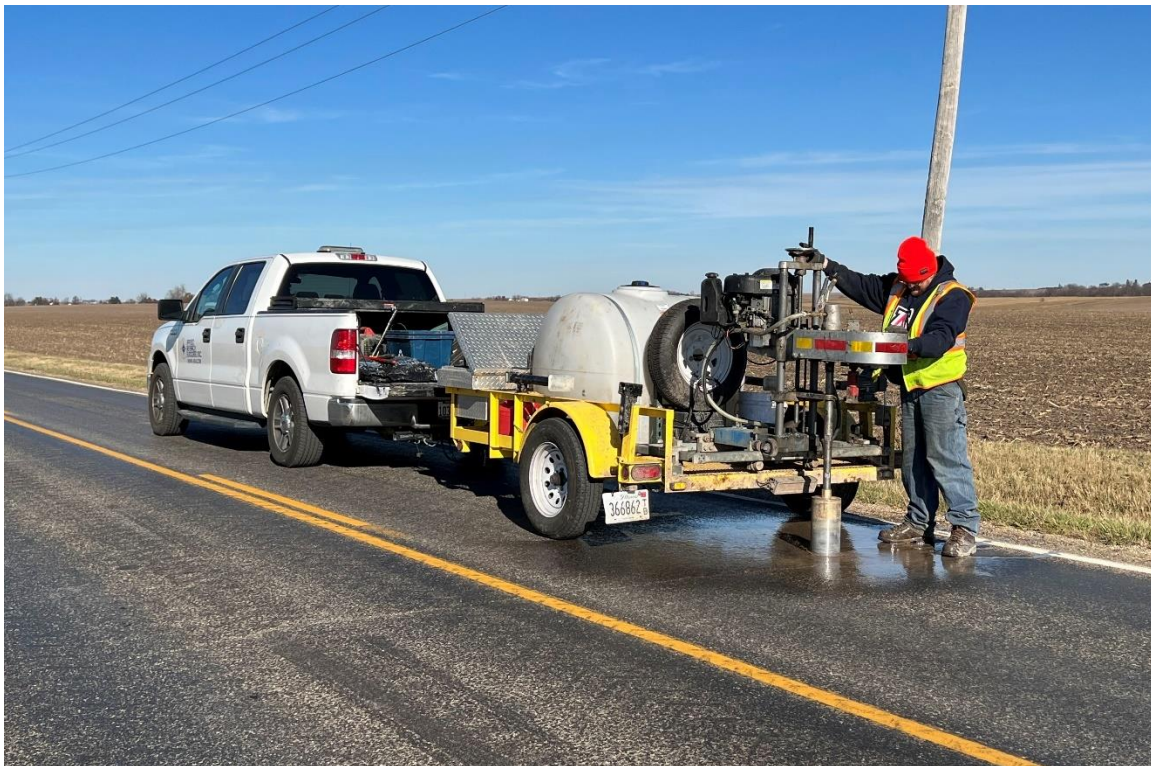
Figure 3. Pavement coring and augering determined the layer types and thicknesses.
