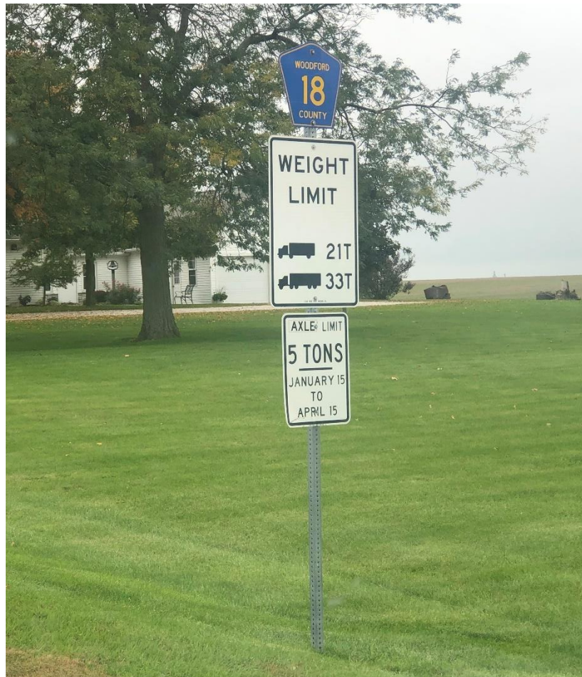
Figure 1. Typical load restrictions on a Woodford County highway.
