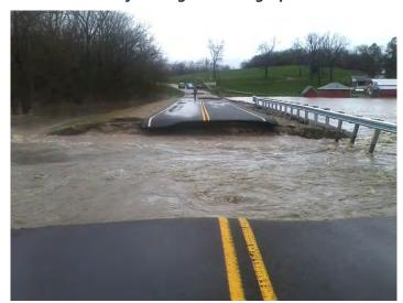
Figure 5.4 - Bartholomew Roadway Damage following Upstream Dam Failure, 2013
