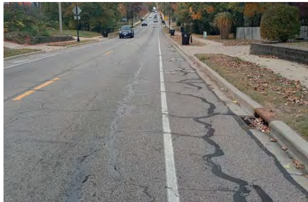
Example of a bike lane on Forrest Hill Ave.
