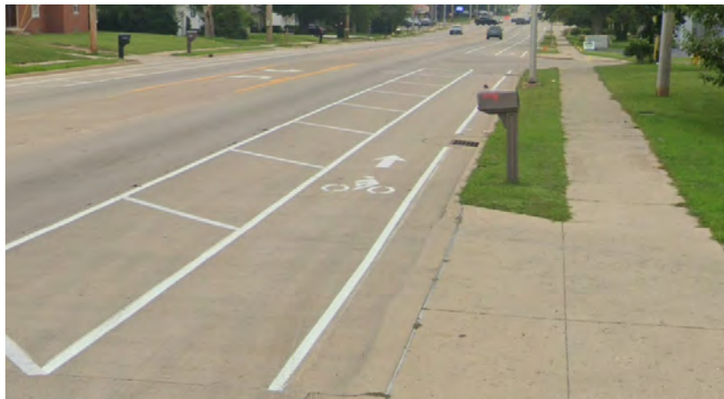
Lower cost roadway reconfiguration to add buffered bike lane on Forrest Hill Ave.
