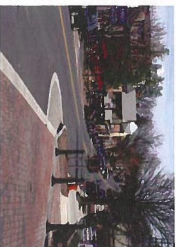
Quick build barriers protect pedestrians in crosswalk from left turning traffic
