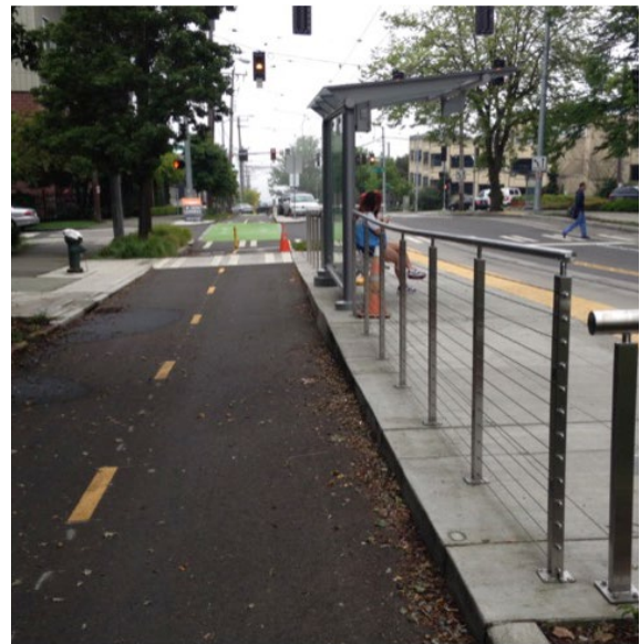
Example of a floating bus stop island and separated bike lane channel that reduces conflicts between bicyclists and buses (source: Dongho Chan)
