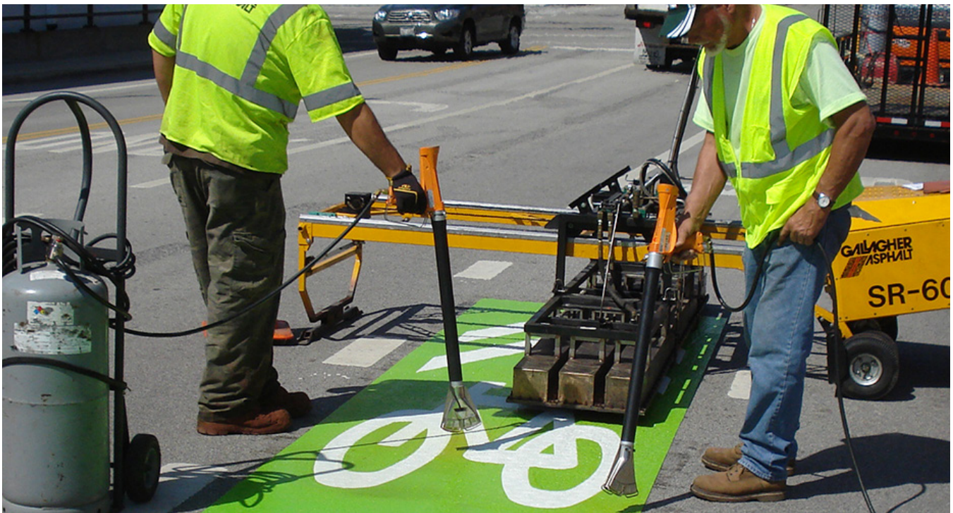
Maintenance crew installing green-backed shared lane markings. (Source: City of Chicago, IL)
