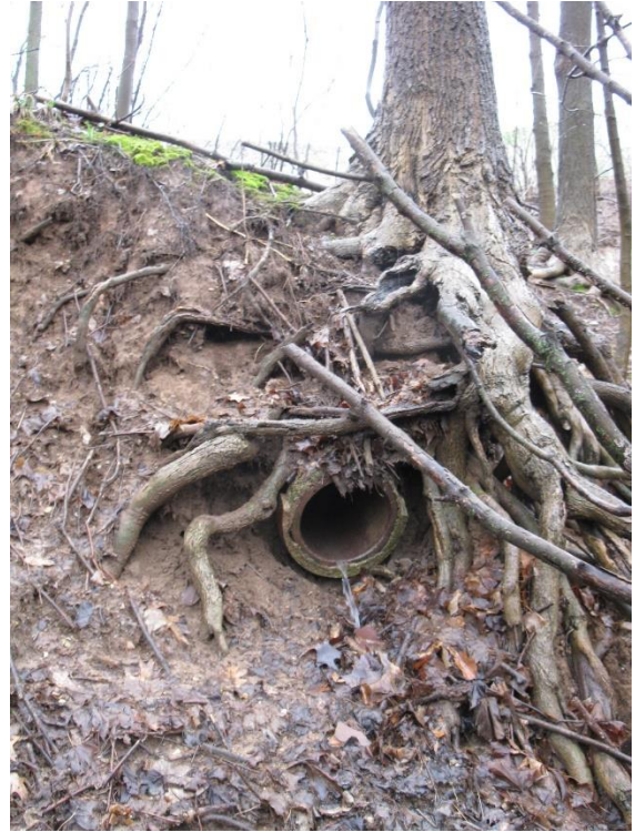
Figure 73: Old Drainage Tile
