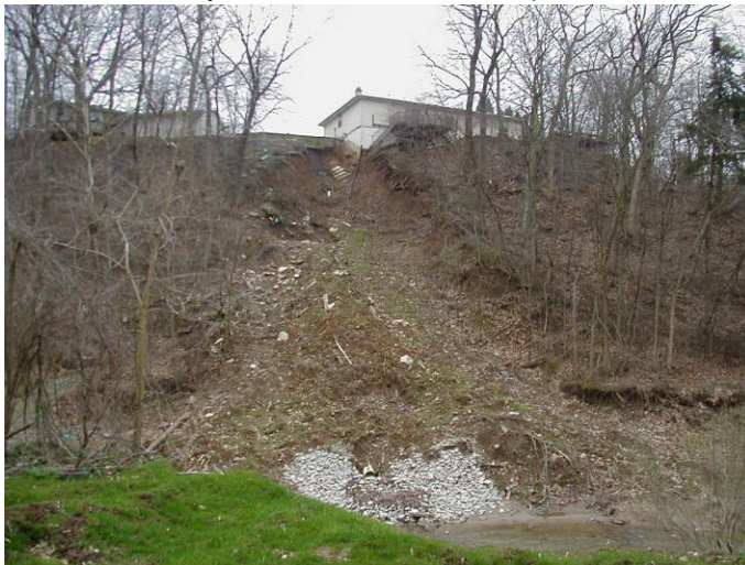
Figure 95: Example of a Failed Slop Near a Municipal Storm Drain Outlet
