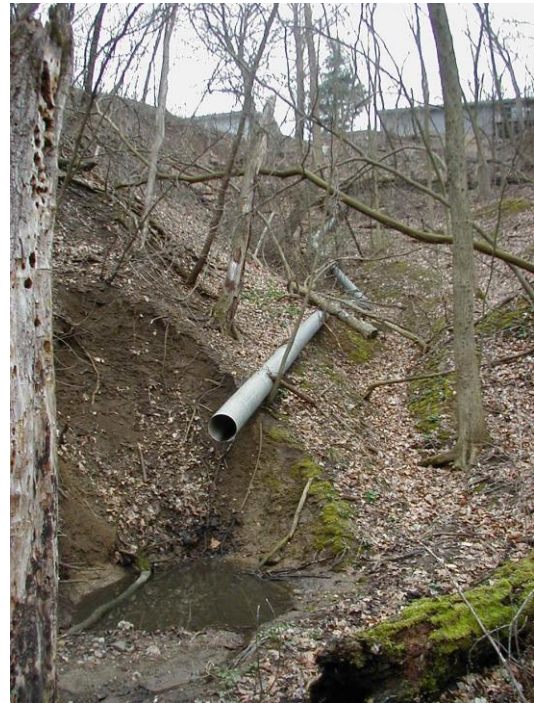
Figure 96: Failed attempt to manage ravine gully erosion from residential area stormwater runoff
