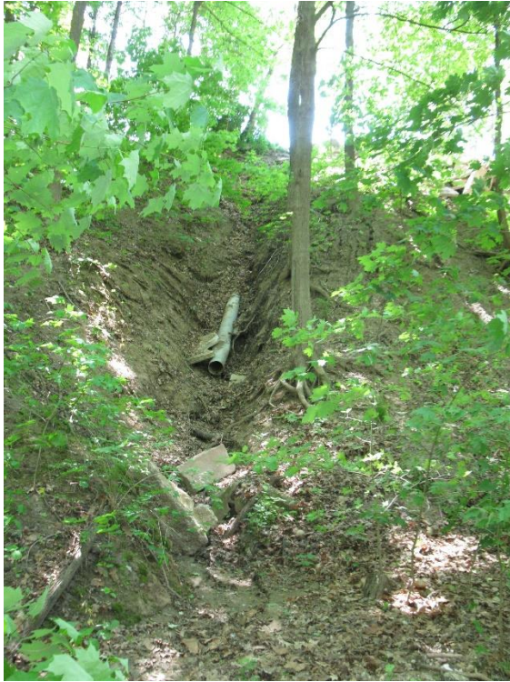
Figure 74: Steep Slope Erosion
