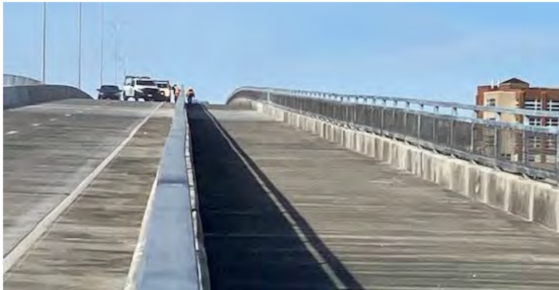
Figure 32: Bob Michel Bridge Almost Finished 12/16/23. Photo Credit: Ray Lees
