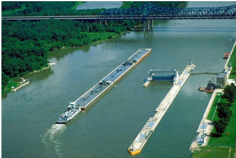
Figure 58: Peoria Lock and Dam During High Flow and the Wicket Gates Down (Peoria Lock and Dam)
