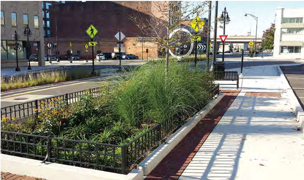
Figure 42: Bio-Based Stormwater Infrastructure (Bioswales) in Downtown Peoria
