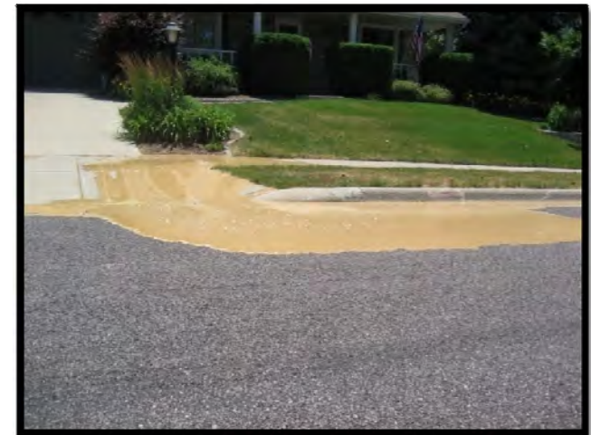
Figure 17: This utility maintenance activity in the City of Peoria created silt that emptied directly into a local stormwater inlet.
