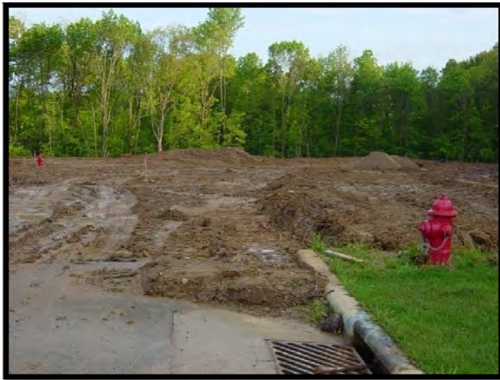
Figure 18: No erosion control combined with extensive soil disturbance at this East Peoria development site created potential for massive soil loss and siltation.
