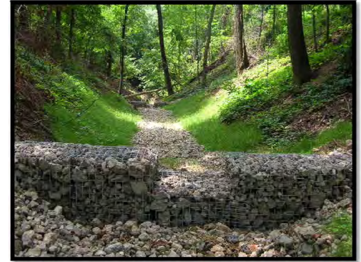
Figure 25: This Mossville Bluffs outlet was stabilized with rock gabion baskets and rock lining.
