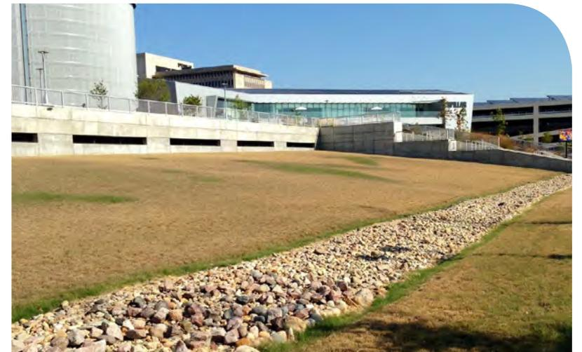
Top Left: Stormwater runoff can cause flooding when proper precautions aren't taken. Top Right and Bottom: The Peoria Riverfront Museum has used native landscaping, bioswales, and a riparian buffer to minimize stormwater runoff.
