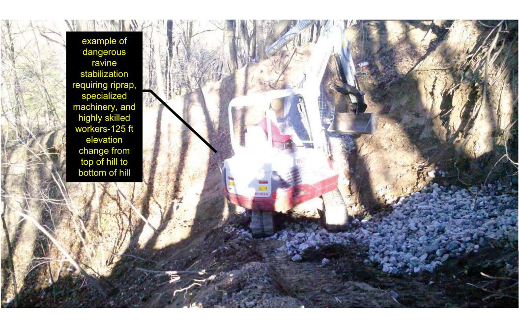
example of dangerous ravine stabilization requiring riprap, specialized machinery, and highly skilled workers-125 ft elevation change from top of hill to bottom of hill
