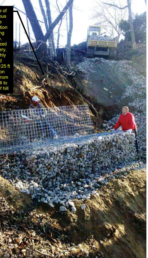
final product of ravine stabilizationnearly 250 tons of riprap
