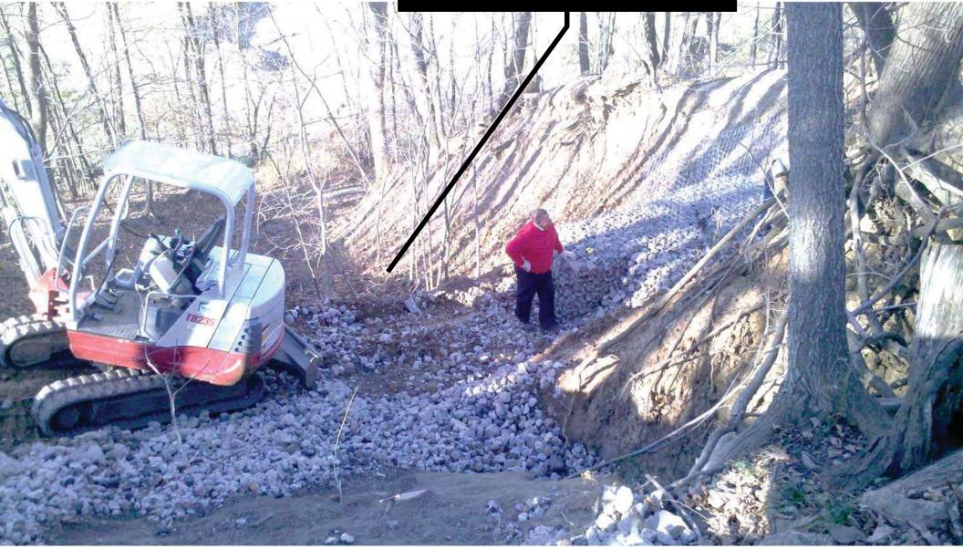
example of dangerous ravine stabilization requiring riprap, specialized machinery, and highly skilled workers-125 ft elevation change from top of hill to bottom of hill
