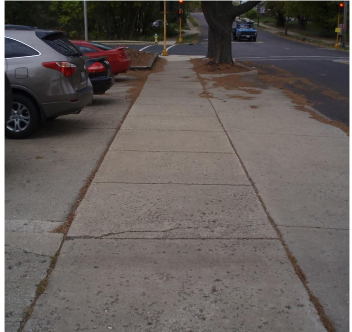
Figure 8. Minor Spalling and Cracking of a Sidewalk.
