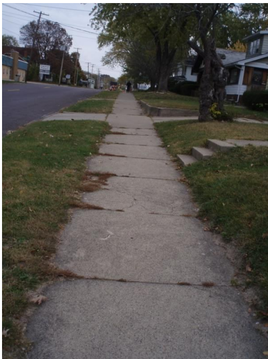
Figure 17. Sloped and Broken SW.
