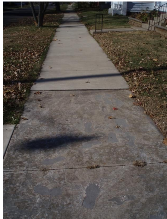
Figure 7. Footprints Poorly Patched.
