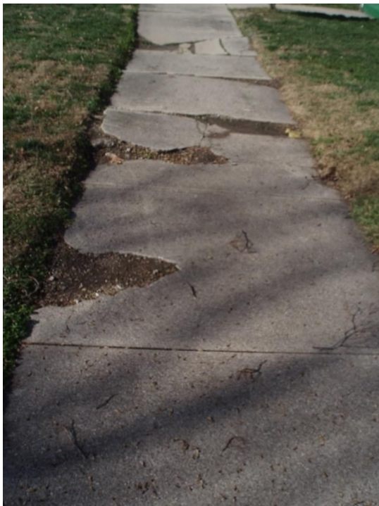
Figure 13. Half of Segment Destroyed (Other Half is Good).
