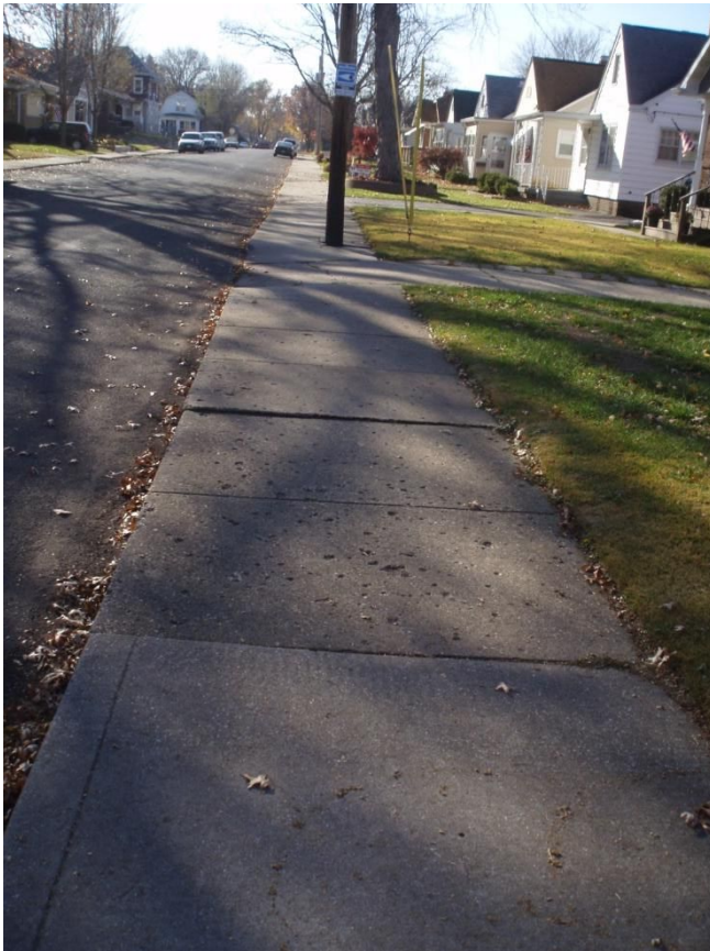
Figure 15. Vertical Lift with Spalling and Cracking.
