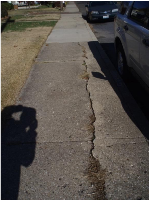
Figure 24. Major Crack with Vertical Lift Thru Entire SW.
