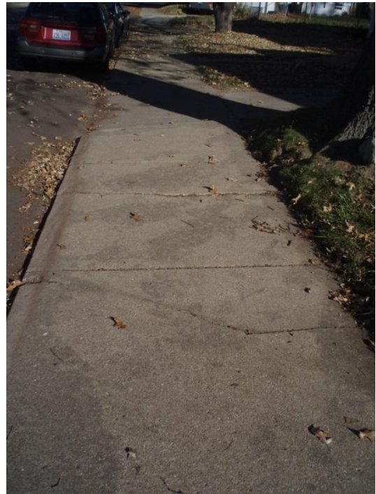
Figure 12. Cracks and Footprints in SW Segment.
