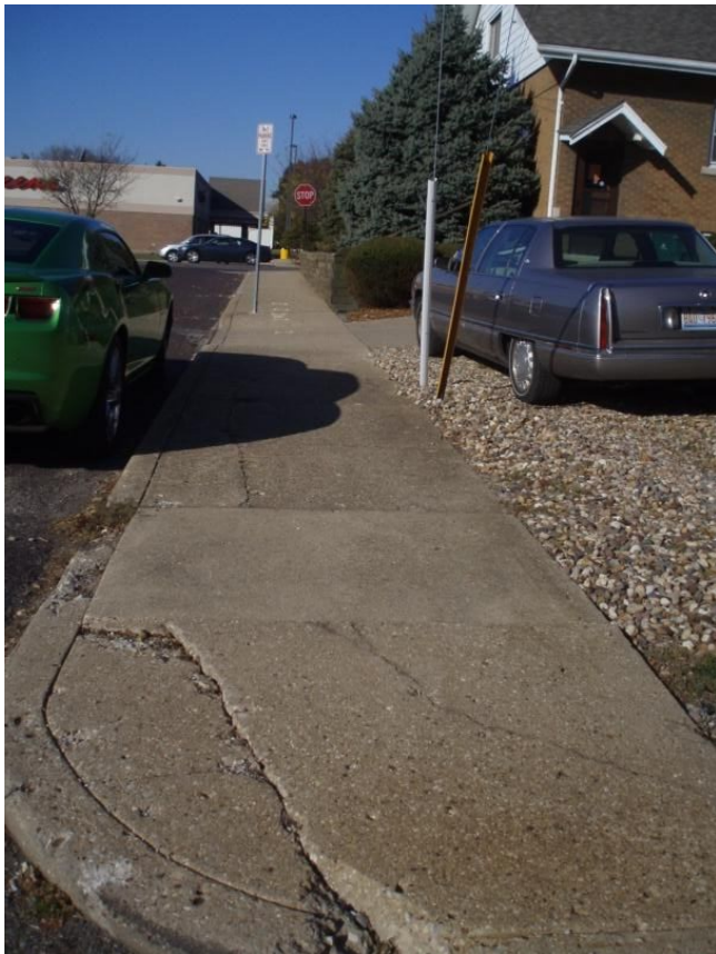
Figure 22. Crack Through Almost Whole SW.
