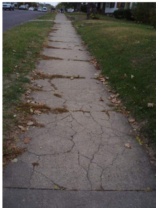
Figure 18. Completely Broken SW.
