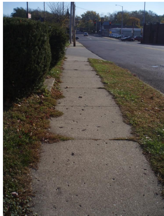
Figure 5. Cracking and spalling
