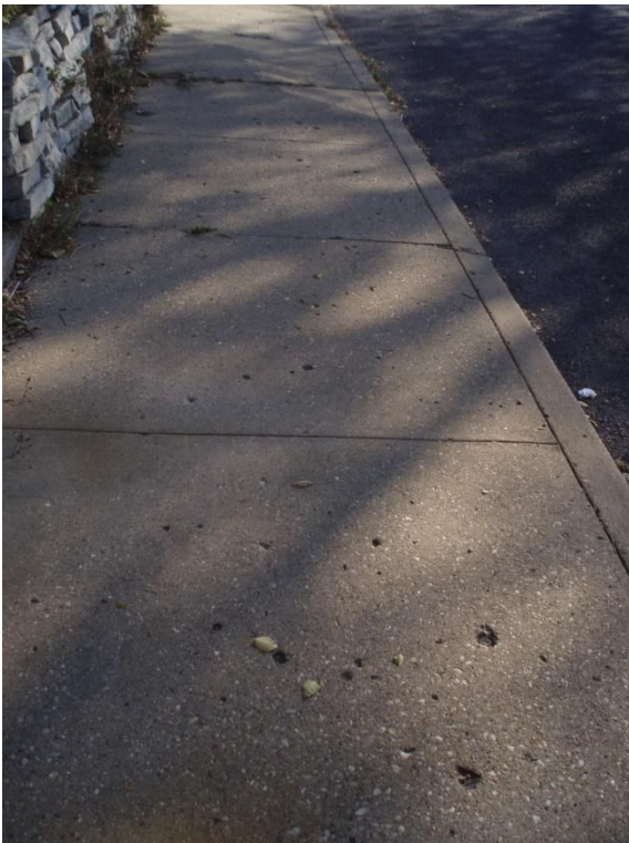
Figure 3. Minor Spalling.
