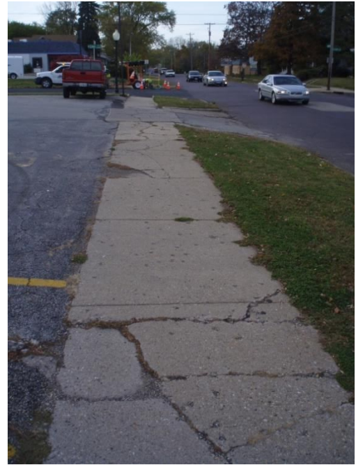
Figure 21. Nearly all of SW Broken/Cracked
