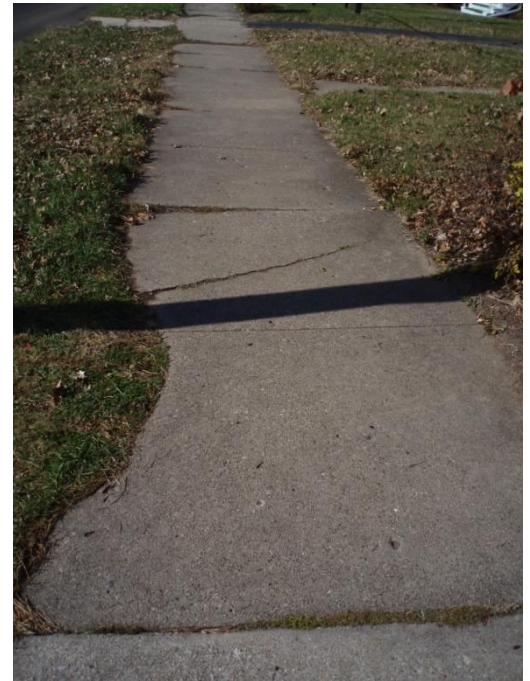
Figure 11. Vertical Lift in SW
