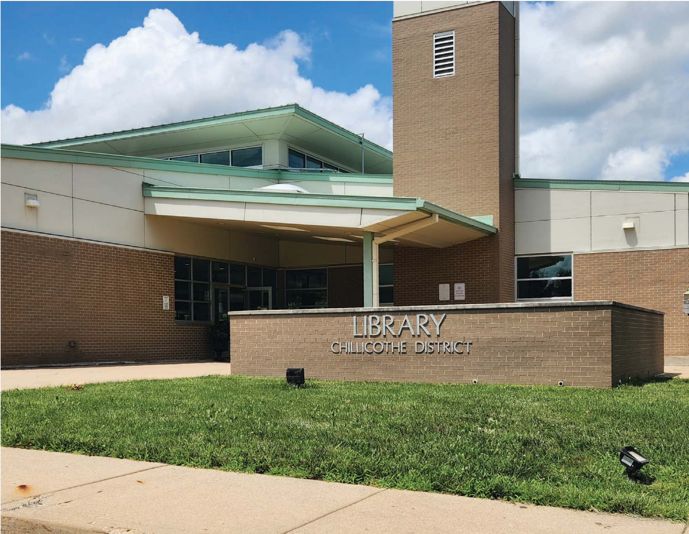
Fig. 1.47 (Right) Chillicothe Public Library District entrance.
