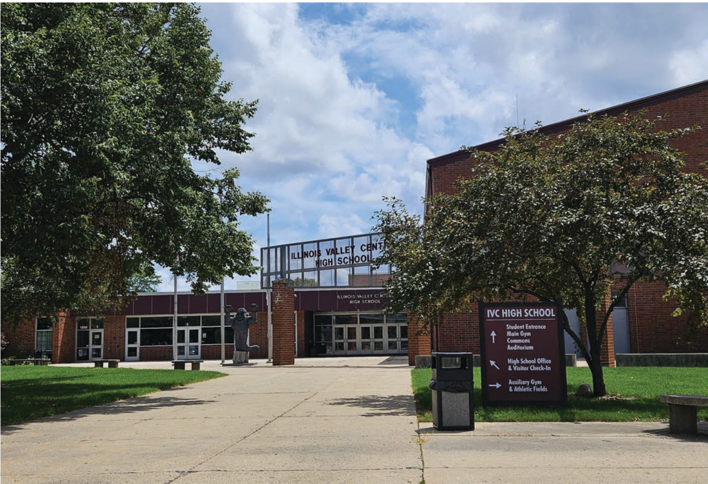
Fig. 1.46 (Below) Illinois Valley Central High School.
