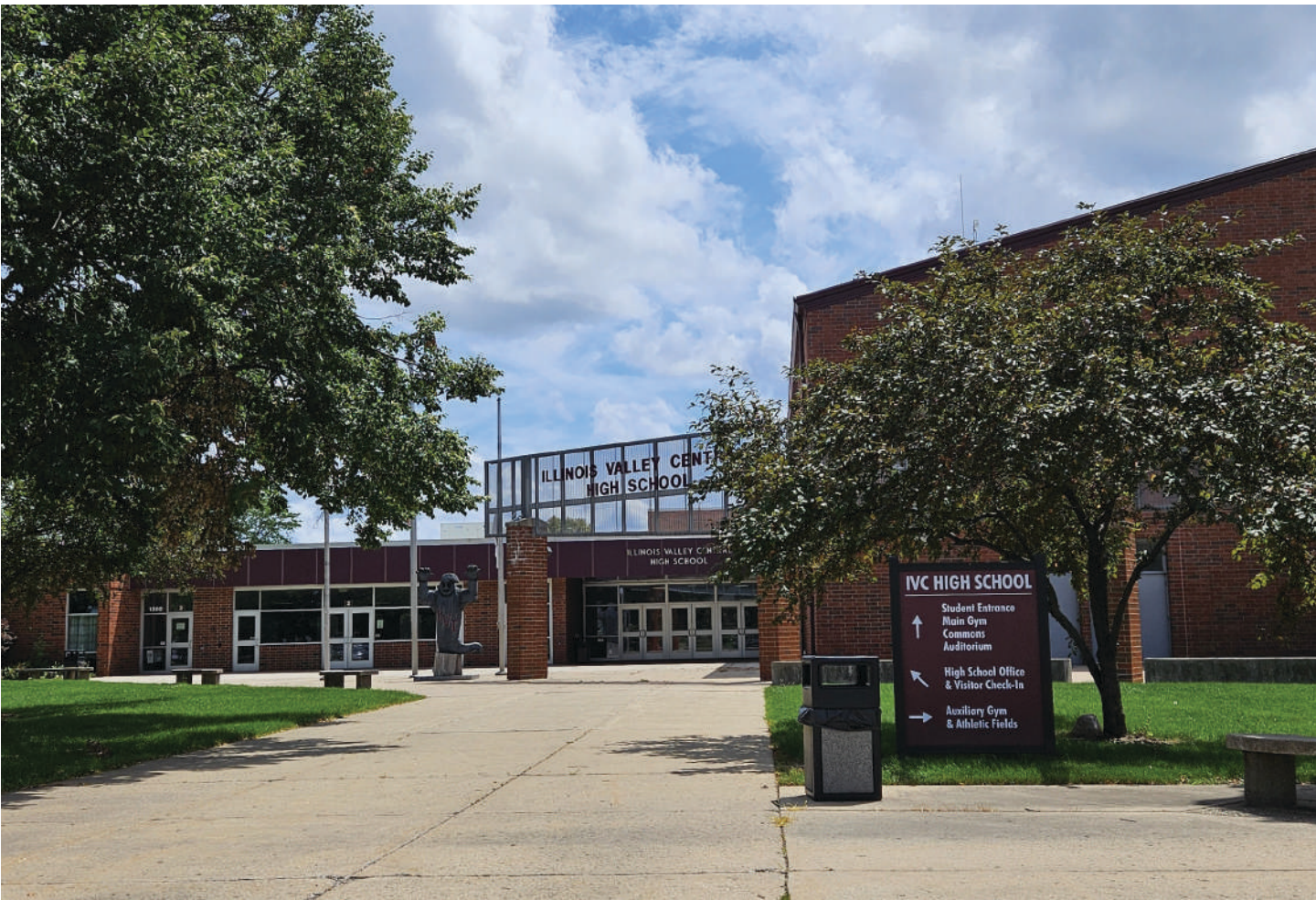
Fig. 1.46 (Below) Illinois Valley Central High School.
