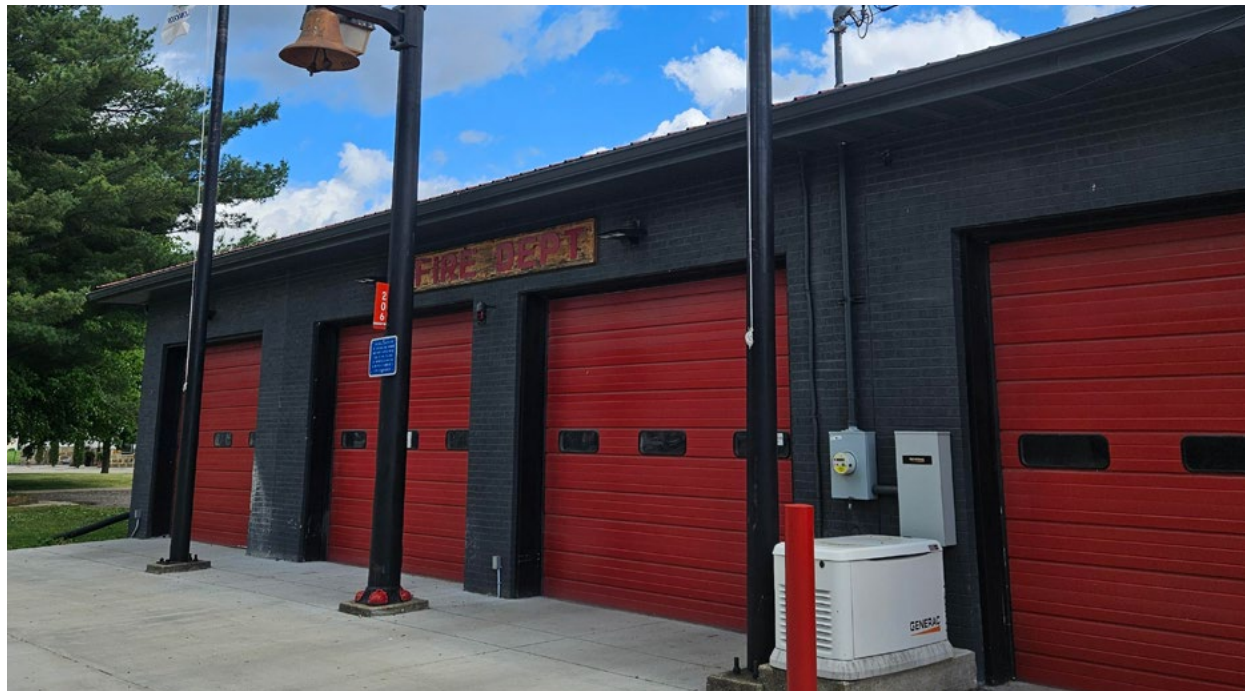
Fig. 1.20 (Above) The Brimfield Community Fire Protection District.
