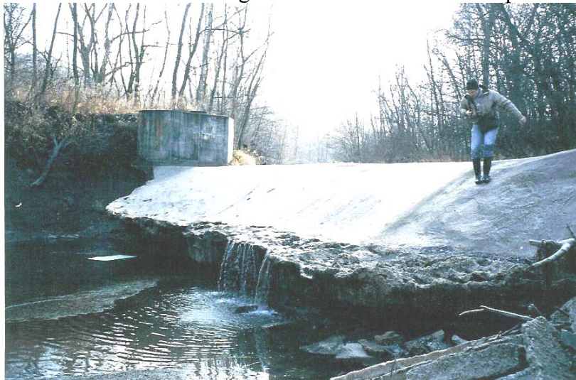
Concrete protection placed over City of Morton sanitary sewer pipe (circa 1980)
