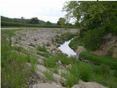
Ackerman Creek along Veteran's Rd: While the left bank is stabilized with riprap, the opposite side of the creek is eroding.
